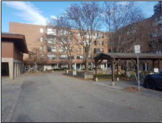
Figure 50: View of courtyard from the parking lot; photo taken November 12, 2020.
