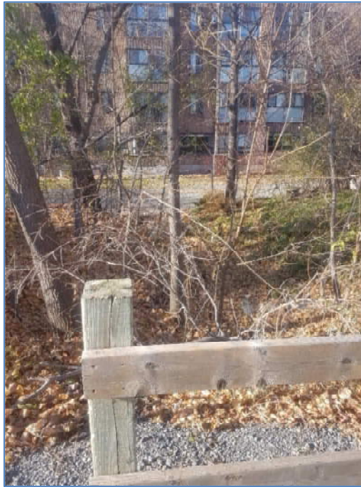
Figure 11: Downstream portion of the first surface drainage feature, south of the Unitarian House, facing north; photo taken November 12, 2020.
