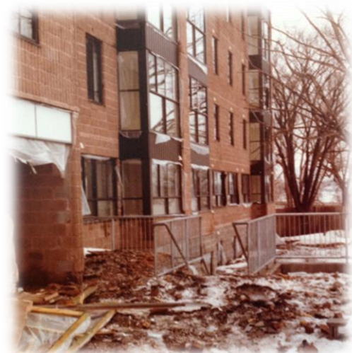
Unitarian House Construction 1984
